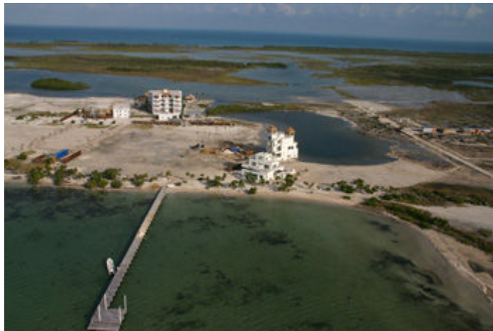
Low lying developments including this one in Belize are prone to damage from hurricanes and high water. They will also be the first to be affected by the rising seas associated with climate change. Lee Pagni/LightHawk
