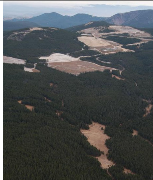
A bald patch interrupts the forest surrounding the Luttrell Pit area which buzzes with activity during the summer months with construction vehicles moving contaminated soil into the repository pit. Less than two miles from the pit, a roadless area provides safe passage for wildlife. Peter Ponca/LightHawk
